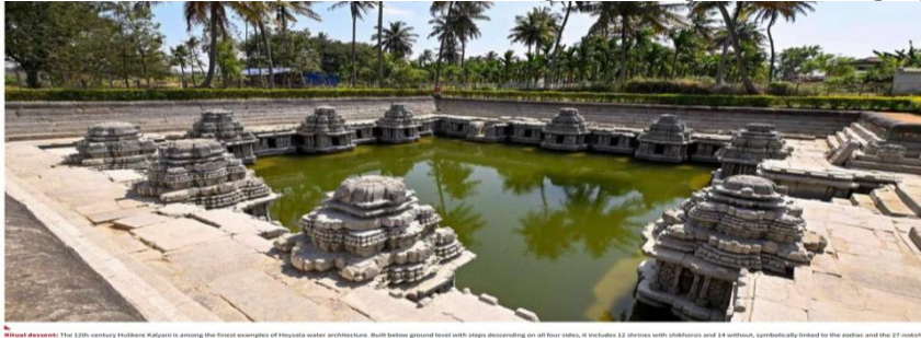
Photo courtesy: The 12th-century Halebidu Kalyana is among the finest examples of Hoysala water architecture. Built below ground level with steps descending on all four sides, it includes 12 shrines with shrines and 14 carvings, symbolically linked to the earth and the 27 constellations.
